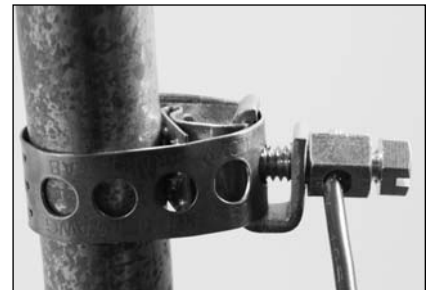
Step 3 - Insert Wire Into the Bolt Hole
