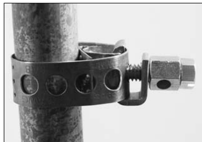
Step 2 - Insert Bolt Through Both Copper Holes
